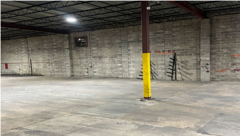
Existing condition - masonry warehouse
