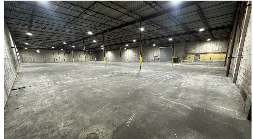
Existing condition - dock & grade-level loading
