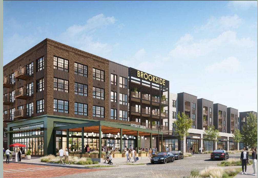
LUXURY APARTMENTS | 335 UNITS
